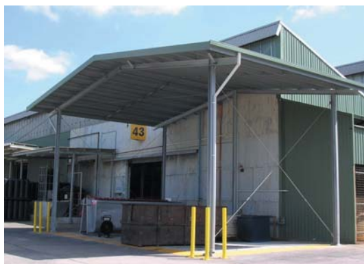
Scrap bins are now located in one bunded area.
